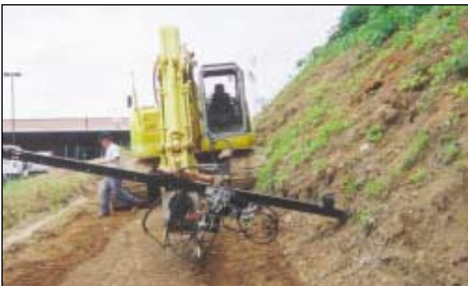
ANCHOR DRIVER MACHINE ON EXCAVATOR
